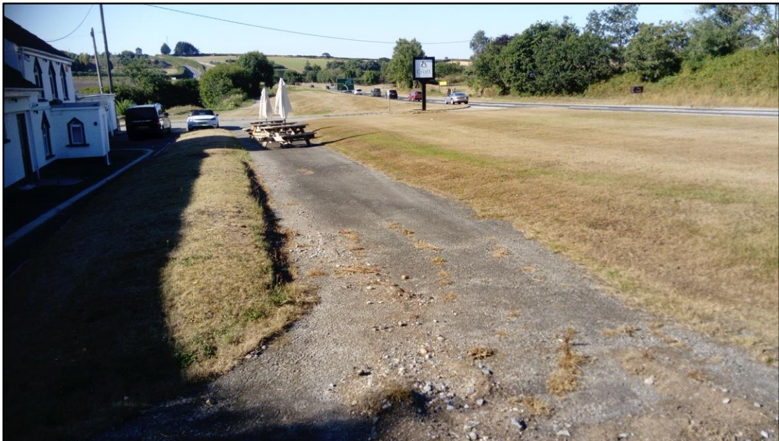
Figure 4.5. Existing bitmac surfacing in front of The Croft Inn
